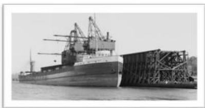
Freighters At Copper Range Coal Dock-1906
